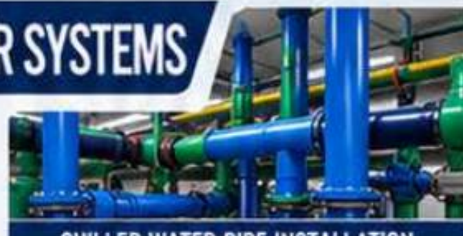
CHILLED WATER PIPE INSTALLATION
